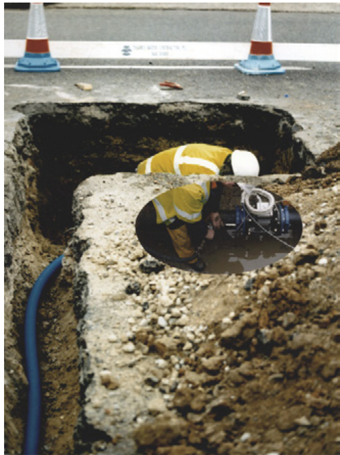
Underground Installation of AquaMaster R
