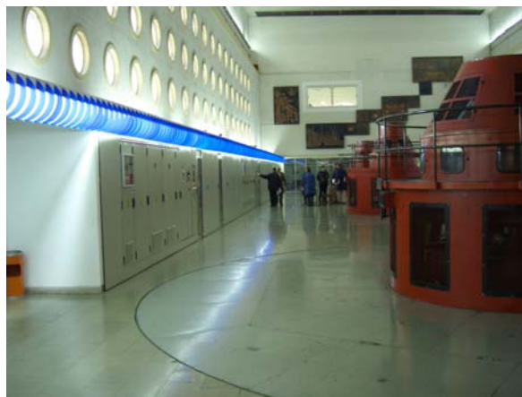
Turbine hall after completion of the upgrading measures
