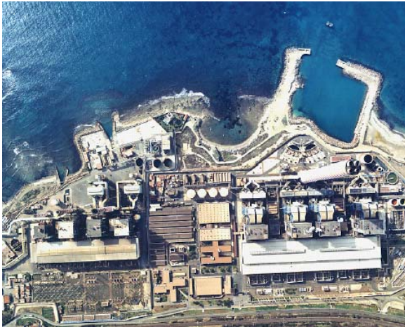
Aerial view of Torrevaldaliga Nord
