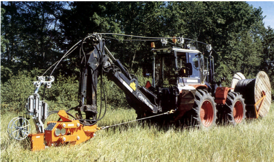
Fig. 2 Ploughing of cable, normally at a depth of 50-70 cm.
