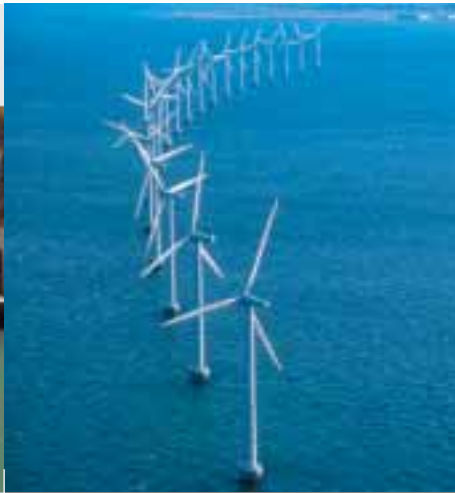
Grid connection of wind parks
