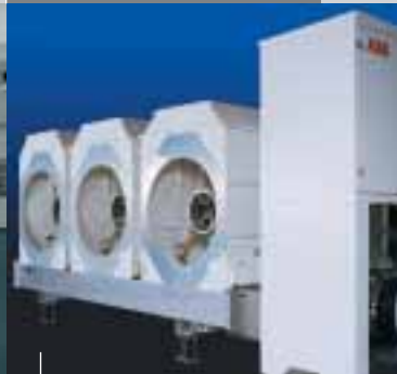
Generator circuit breaker
