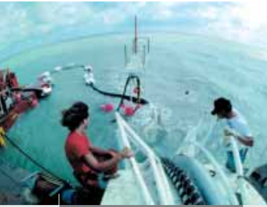
Laying of submarine cables
