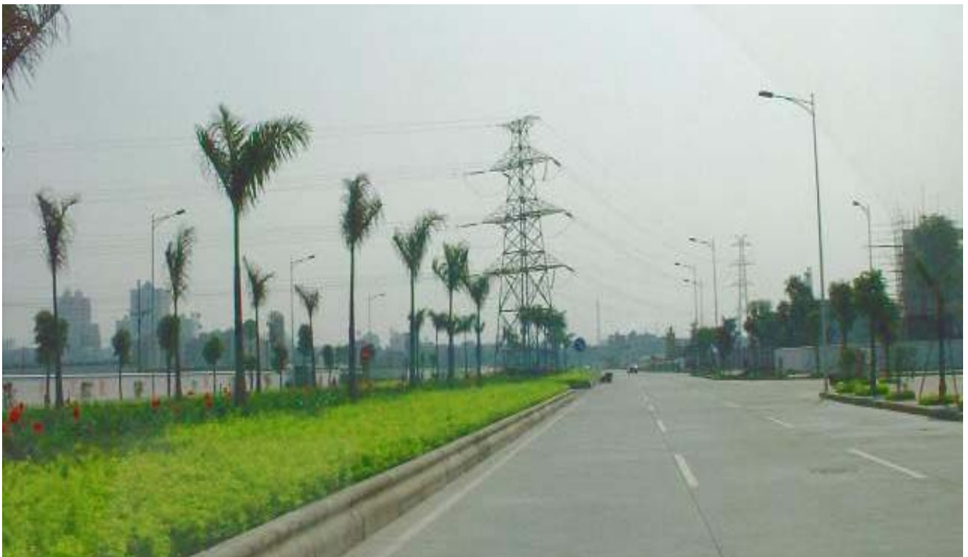
In a cablification project in the city of Guangzhou (Canton) ABB replaces the overhead lines with cables.
